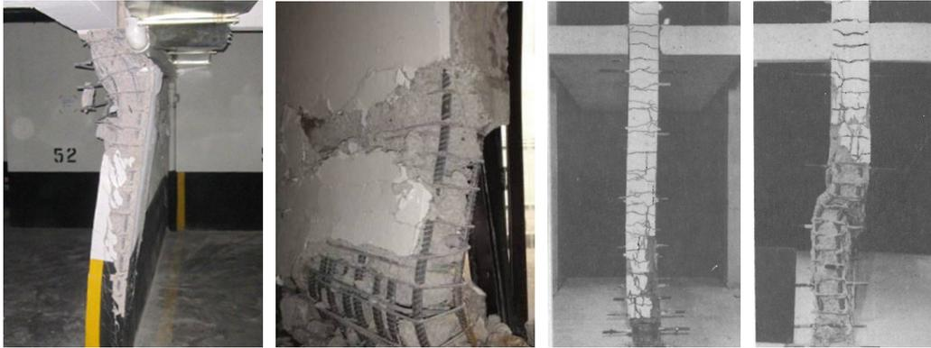
**Figure 3.1.** Examples of overall wall buckling: (a) 2010 Chile Earthquake (photo by Professor Jack Moehle) (b) 2011 Christchurch Earthquake (Kam et al 2011) (c, d) Tests by Goodsir (1985)
