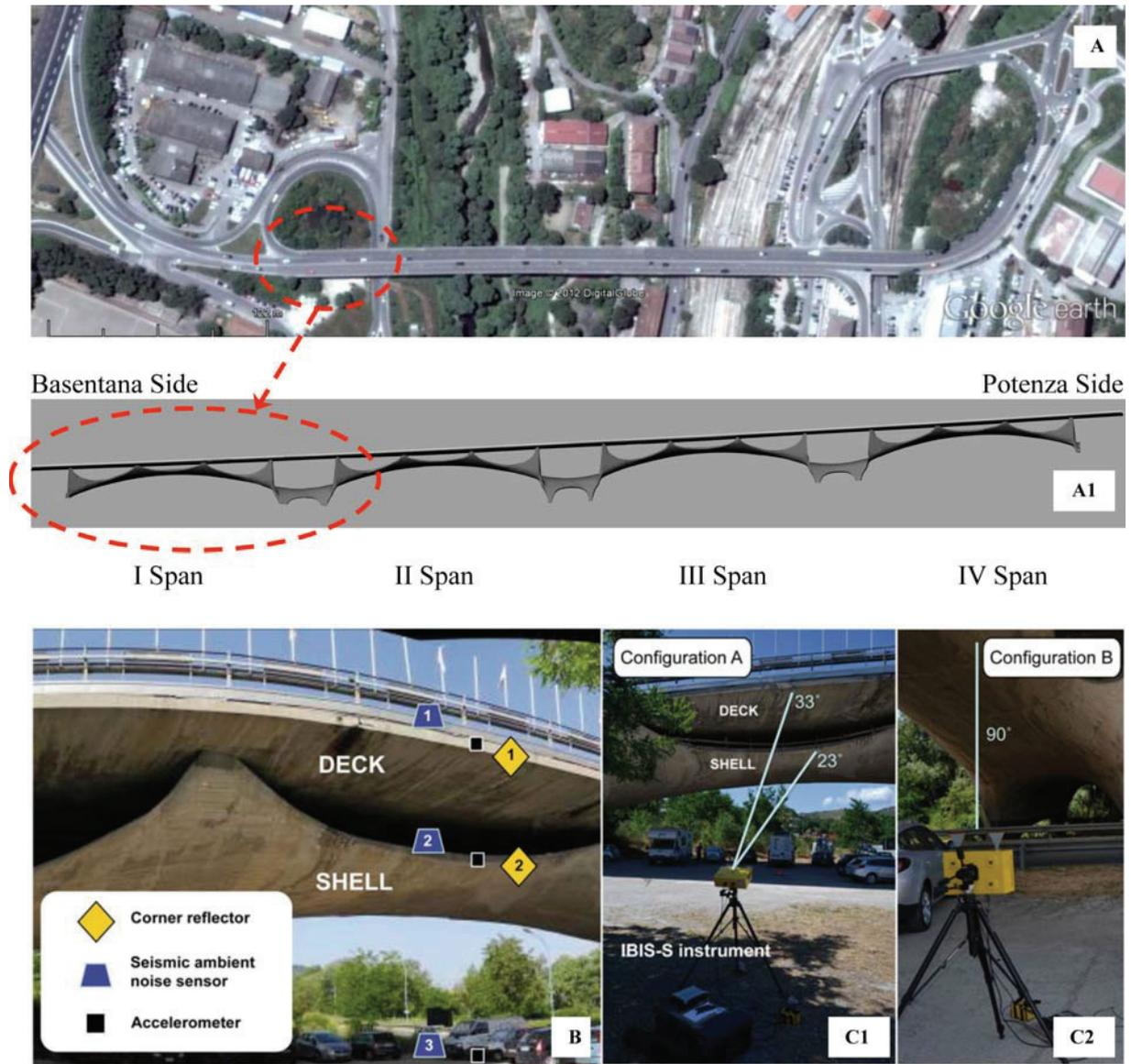
**Figure 4:** (A) Plan and (A1) sketch of the section of reinforced concrete Musmeci bridge; (B) Sensors installation at the Musmeci Bridge; (C1) Installation of the IBIS-S system in the configuration A; the sensor was placed in front of the bridge, illuminating the shell and the deck with LOS angles of  $23^\circ$  and  $33^\circ$ , respectively. (C2) Installation of the IBIS-S system in the configuration B; the sensor was placed vertically under the bridge (LOS angle =  $90^\circ$ ).
