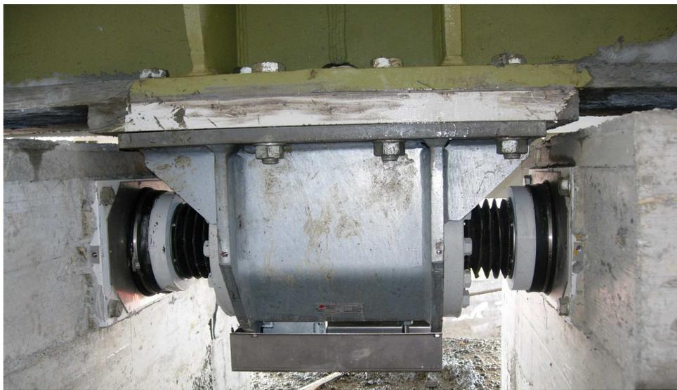
**Figure 5.** OP series viscous dampers installed in transverse direction of the bridge (on P1 ÷ P10 and SP2 positions, see Figure 3).
