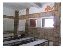
Figure 6: RCC splints and bands on interior walls
