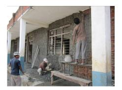
Figure 9. Micro-concreting grouting
