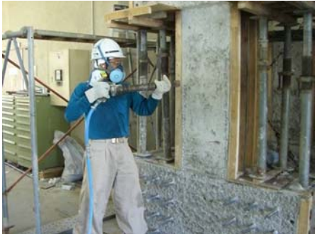
Photo 2.1 Concrete roughening works
