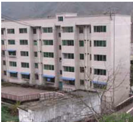
(a) The survived 7 story masonry with first used as shops
