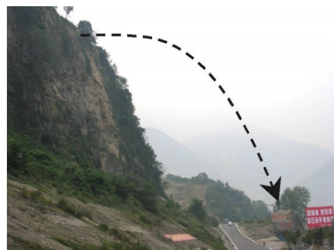
Figure 3.4. 300t rock travelled 60m by catapulting had been found on Duwen Road, Yingxu town [12]
