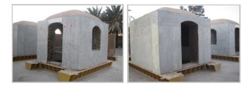
Figure 17. With natural fibre reinforced burnt brick (left) and with natural fibre reinforced mud brick (right)
