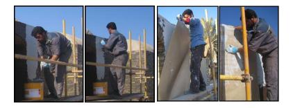
Figure 15. Application of the first adhesive layer with a trowel
