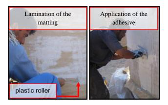
Figure 16. The Lamination of the matting onto the adhesive layer and Application of the adhesive layer on the matting
