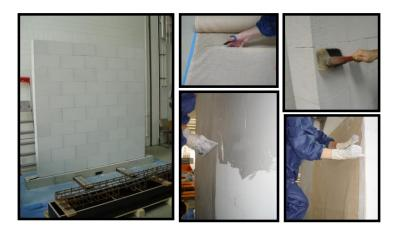
Figure 10. Reinforcement of masonry wall with jute fibre mats
