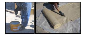
Figure 14. Mixing the two-component adhesive with a mixer (left) and cutting the jute mat to reinforce the walls
