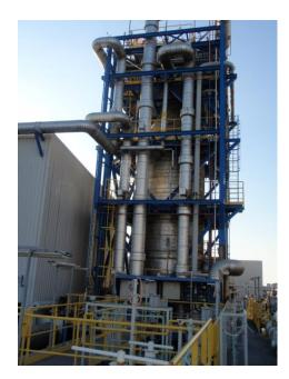
Figure 4 - Steel structure braced for horizontal actions (in blue)
