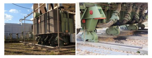
Figure 6 - Power transformer supported on wheels
