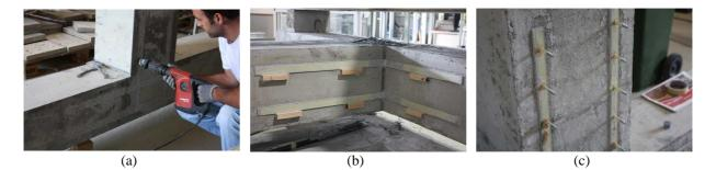
Figure 2.5. Strengthening procedure for the MF-EBR technique: (a) preparation of the concrete surface;(b) MDL-CFRP was placed on the concrete surface by pressing it against to concrete in order to create an uniform thickness of 1 to 2 mm of adhesive layer; (c) application of the anchors
