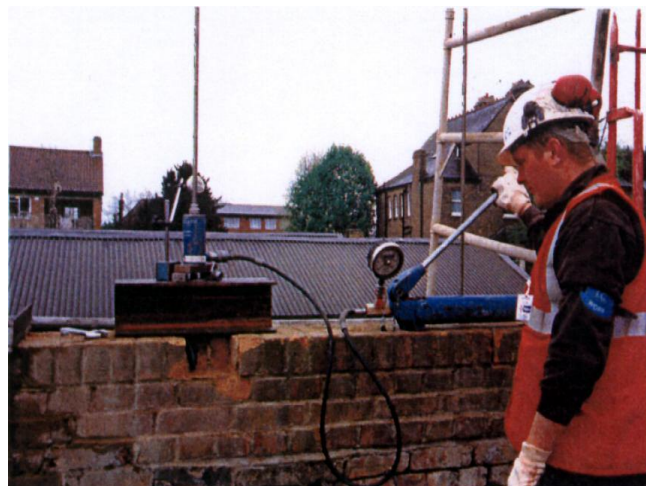
Figure 5. Applying Post-tensioning method
