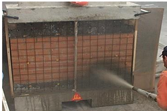
Figure 2. Applying Shotcrete
