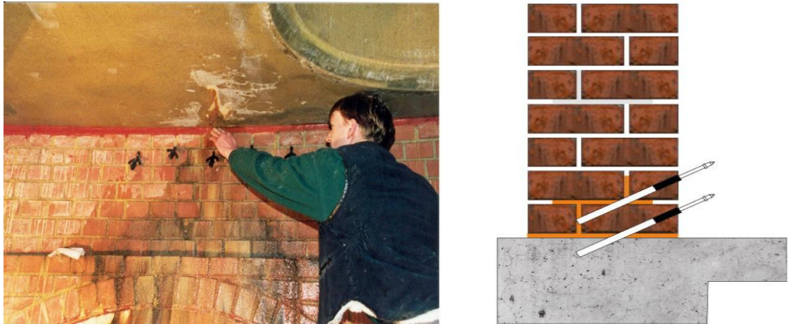
Figure 9. Applying Injection method for existing masonry brick wall
