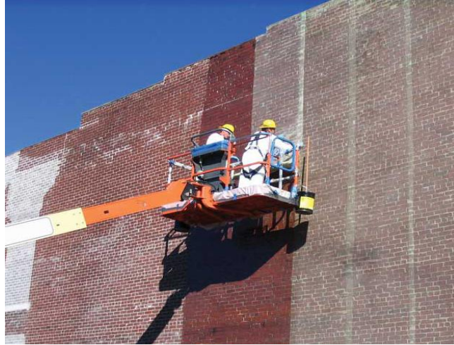
Figure 4. FRP retrofitting method
