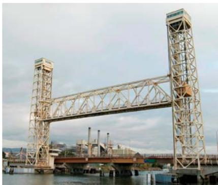
**Figure 1.1.** Fruitvale Railroad Bridge, Lift Span at Mid Position
