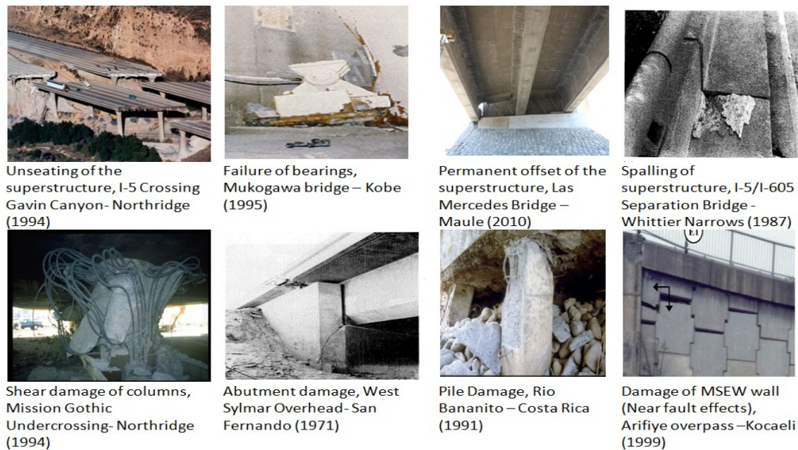
Figure 1. Damage to skewed bridges during different earthquakes
