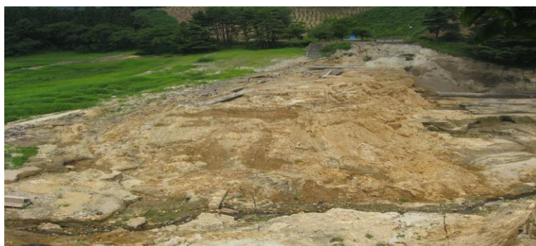
Figure 3. Dam failure after earthquake
