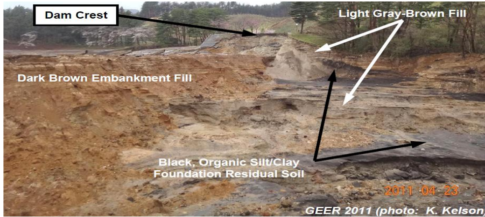
Figure 6. Cross section after earthquake [Harder et al., 2011]
