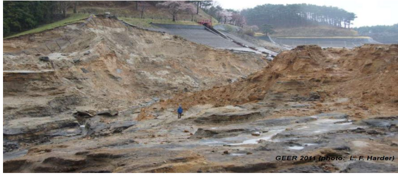
Figure 4. Dam Section after earthquake
