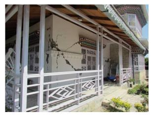
Figure 3. Newly built non-engineered RC house in Sikkim Earthquake 2011
