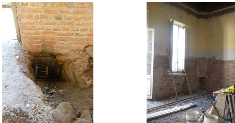
Figure 7. Reinforced foundation beam under wall (left) and cleaning of plaster of masonry (right)
