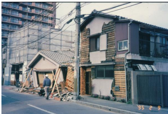
(a) Damage concentrated to the first storey
