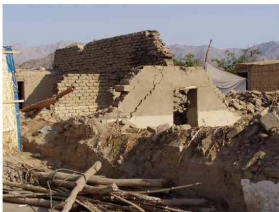
(a) Damaged adobe (2007 Pisco Earthquake)
