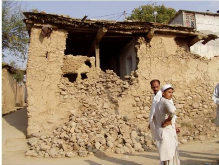
(a) Unreinforced stone masonry
