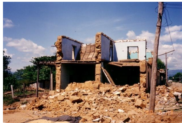
(b) Damaged tapial (1990 Rioja Earthquake)
