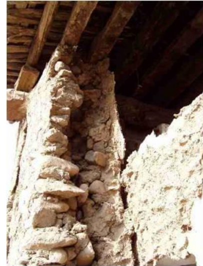
(b) Damage to the stone masonry wall
