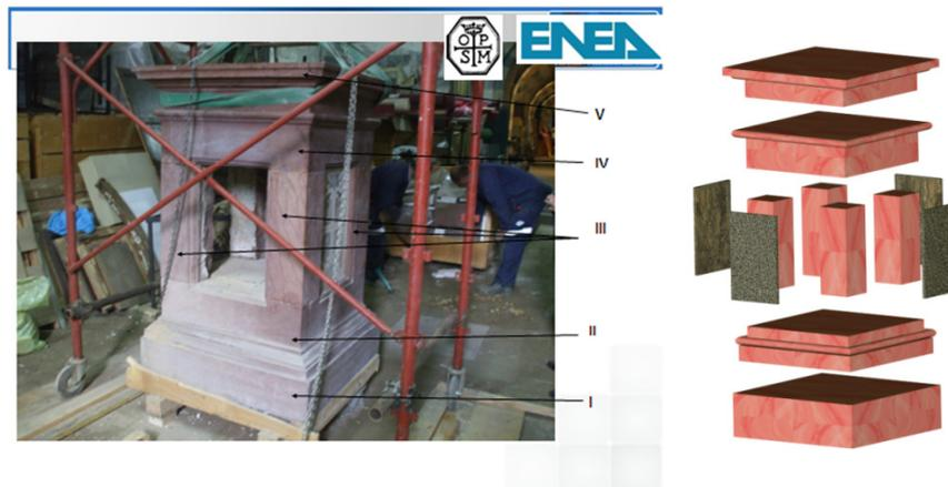
**Figure 17.** original basement of the statues, it is composed by several blocks.
