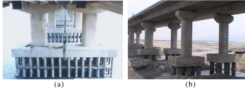
Figure 1.1. Bridge foundation exposure due to riverbed scour (courtesy of (a) Dr. C. Lin and (b) Dr. Y.C. Lin)
