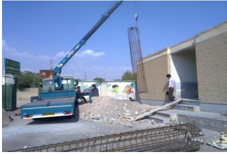
Figure 6: typical retrofitting by shear wall
