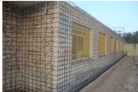
Figure 7: typical retrofitting by peripheral shotcrete
