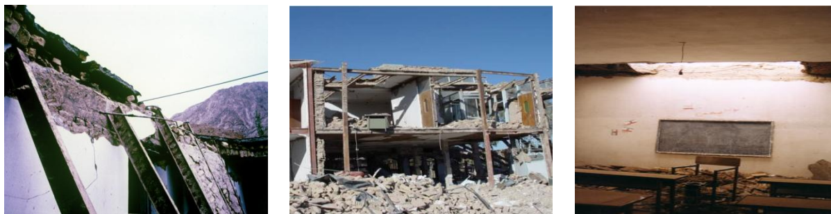
Figure 1: Collapse of jack arch slabs (partial and complete) for lack of integrity
