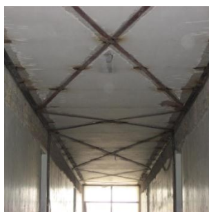
B. Diagonal steel bracing
