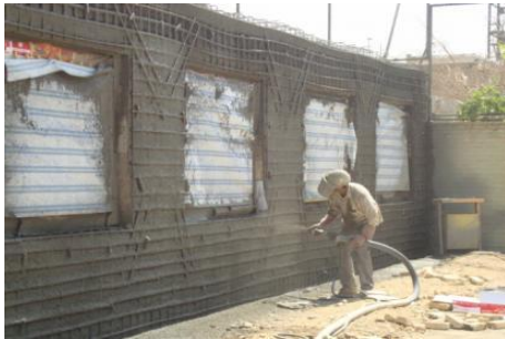
Figure 7: typical retrofitting by peripheral shotcrete
