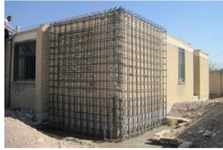
Figure 6: typical retrofitting by shear wall
