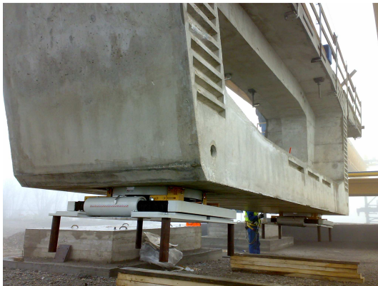
Figure 10. Installation of combined devices in the Oglio bridge.
