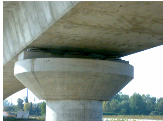
Figure 11. Combined devices and mechanical fuse restraint as installed in the fixed pier of the Oglio bridge.
