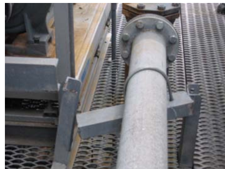
(a) Pipe on the roof
