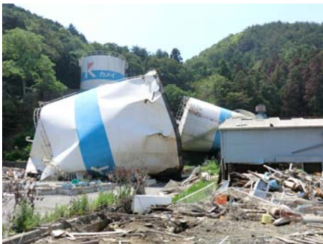
Figure 22. Tanks washed away by the tsunami
