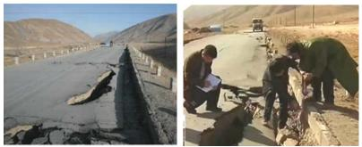
a) Highway foundation settlement and crack
