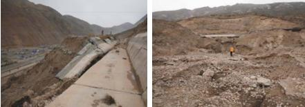
c) Foundation failure of ditch due to landslide d) **Figure 6.** Water-supply damaged due to landslide and active fault
