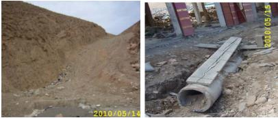
a) Cannel buried by debris or landslide b) damaged pipeline near the active fault
