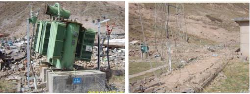
c) Transformer displacement d) snapped electric line Figure 5. Electric power damaged due to strong ground motion
