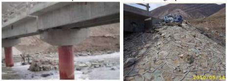
e) Beam displacement and fractured seismic anchor f) cone protection damaged
