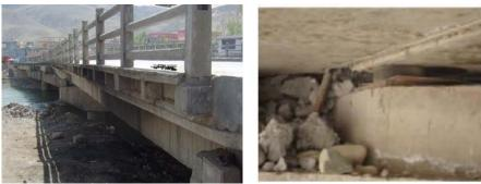
a) Contra rotating and snake motion b) Bearing displacement and fractured seismic anchor
