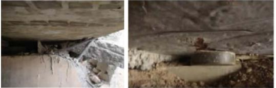
c) Fractured cap beam of abutment d) Baring separation
