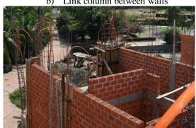
d) Load walls Figure 3. Construction details.
