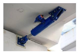
Figure 9. Viscous dampers installed on the abutments PS3 and PS4
