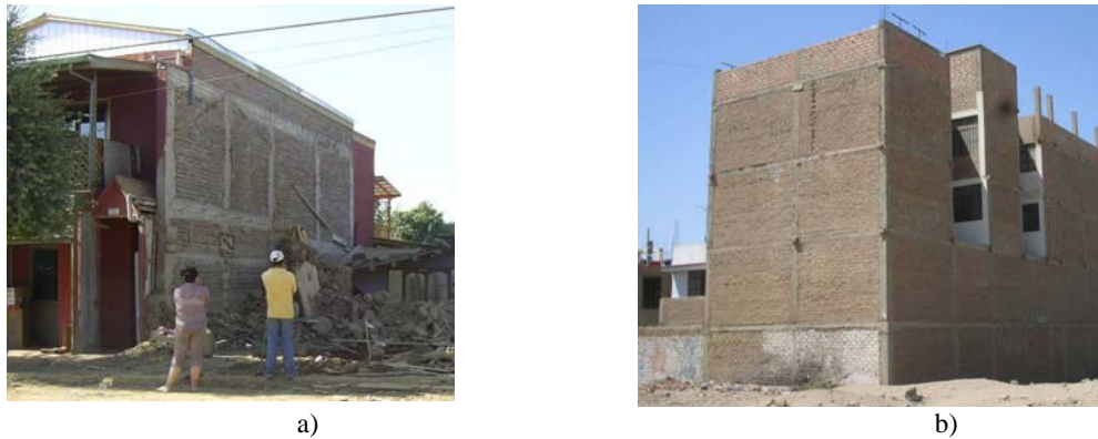
Figure 3. Performance of confined masonry buildings in recent significant earthquakes: a) the 2010 Maule, Chile earthquake (M.O. Moroni Yadlin), and b) the 2007 Pisco, Peru earthquake (D. Quiun)
