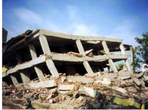
Figure 1.1. Type of Failure Observed in Pre-1970's Building Structures (Izmit, Turkey Earthquake 1999)
