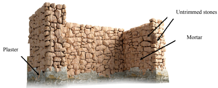
Figure 4.9: Typical external masonry wall
