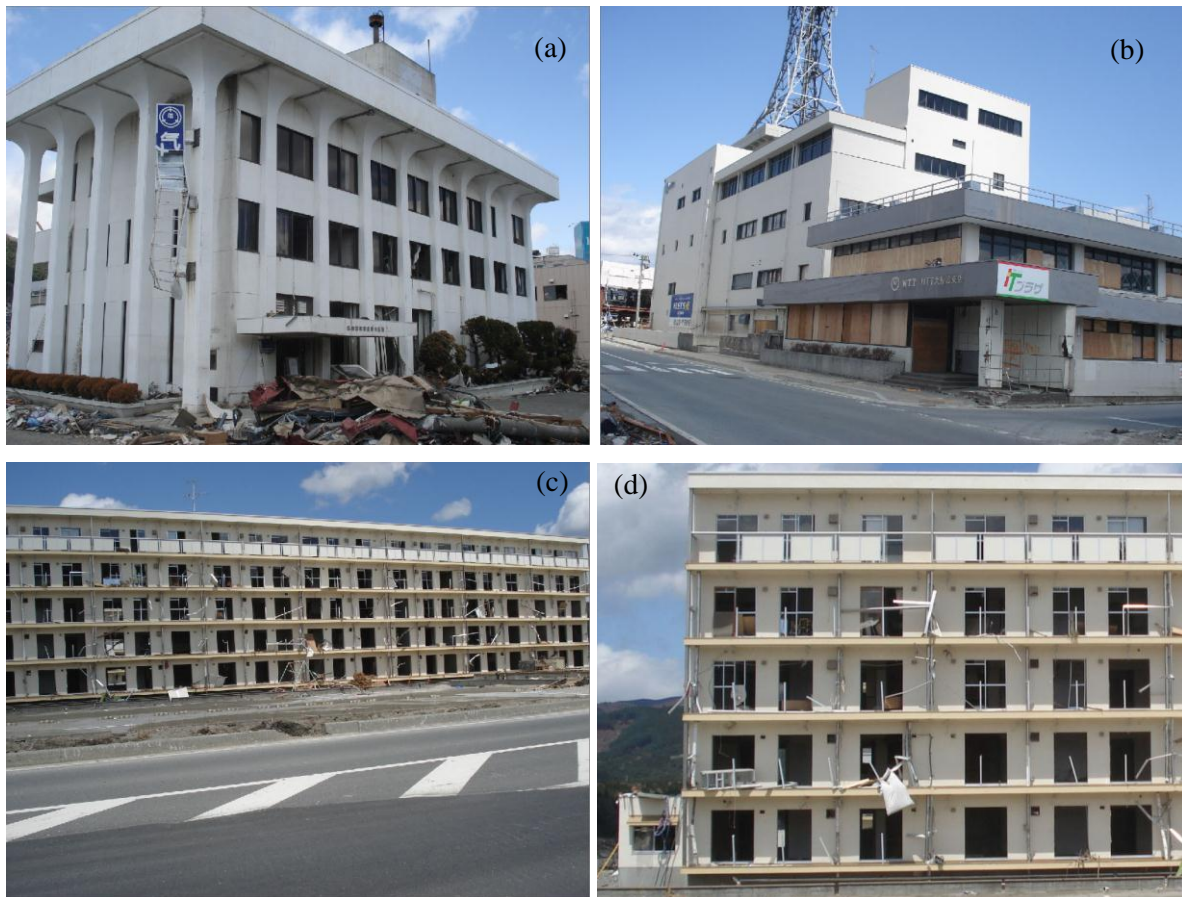
Figure 8. RC buildings after tsunami attack
