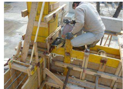
Figure 2.3. HPFRC jacket casting
