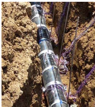
(a) Surveyor's poles for displacements
