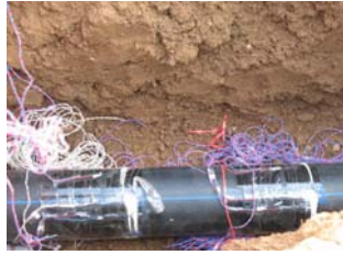
(a) Strain gauges on the pipe
