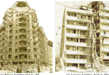
(i) Wilson building built in '30s (ii) Lizeanu building, built in '60s (ii) Collapse of the building soft story at the ground level
