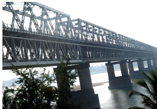
Figure 3.1. Photographic view of the Saraighat bridge.
