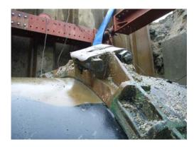
Photo 3.3. Sealing bolt worn out by hydro-blasting
