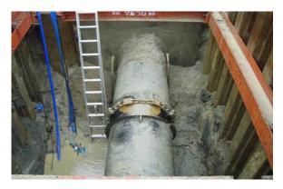
Photo 3.2. Excavation of joint failure portion
