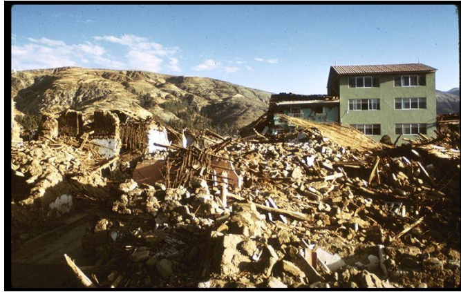
Photo 1 Destruction of adobe houses in Huaraz with a 3-storey reinforced masonry building surviving the shaking (Source: NISEE – The Earthquake Engineering On-Line Archive)
