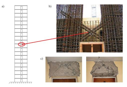
Figure 1.1 a) Schematic of RC coupled wall structure, b) Typical reinforcing detail for diagonally reinforced coupling beams (Wallace 2006), c) Coupling beam damage in recently-constructed high-rise condominiums after Conception 2010 (LATBSDC 2010)
