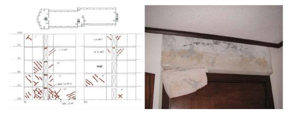
Figure 2. Typical shear wall elevations with crack mapping (left) and damaged link beam (right)
