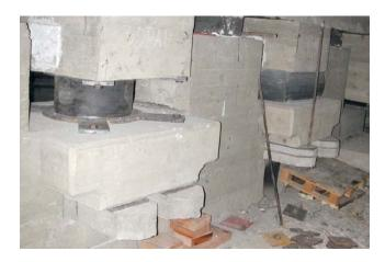
Figure. 1 Installed new and old bearing
