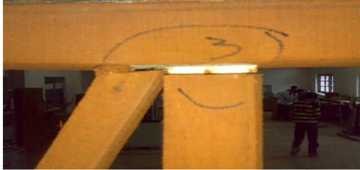
Figure 3. Joint failure at the top of Frame 1
