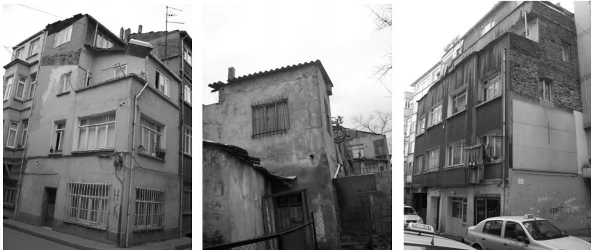
**Figure 4. 3.** Examples of URM buildings in Fatih sub-province with relatively high seismic risk ( $VS > 0.7$ ) after vulnerability score assignment
