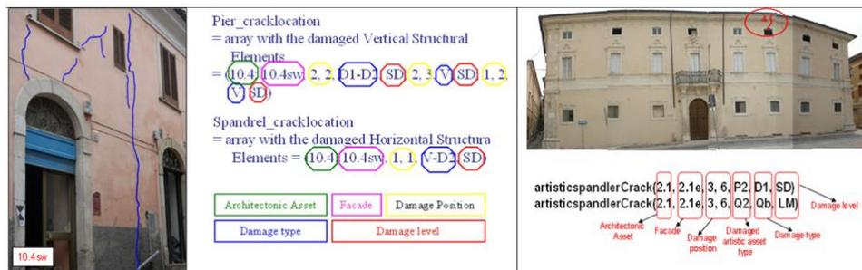
**Figure 4-2** a): Damage identification for the SEs of the façade 10.4sw and b) damage identification for the aas of the façade 2.1e
