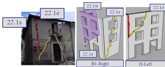
Figure 6-3: LOG-IDEAH Output applied to the façade 22.1e and façade 22.1s
