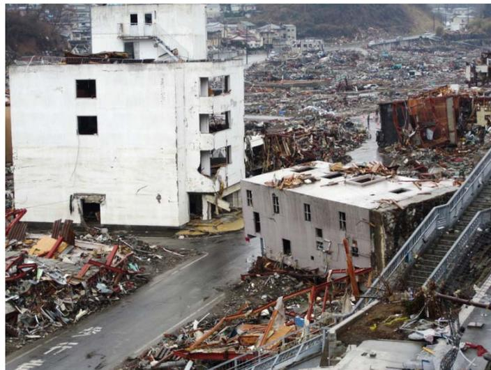
**Figure 8.** Overview of overturned four-story reinforced concrete building C with pile foundation
