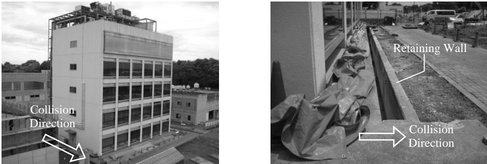
Photo 2.1. The Base-Isolated Building, which is Subject of the Experiment Left: View of the Building, Right: Retaining Wall
