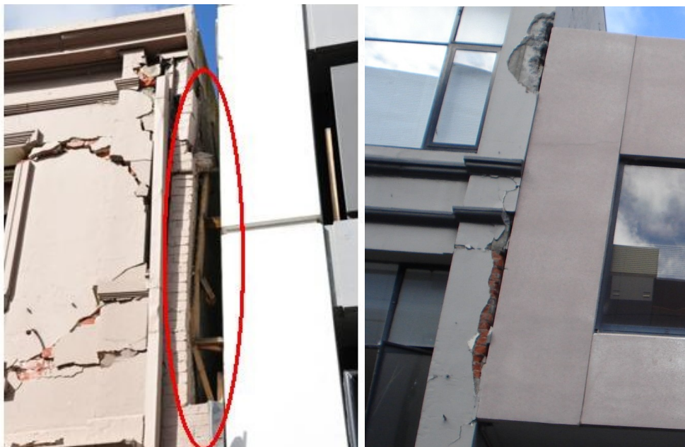
Figure 2.3 Left: Building damage caused by framed flashing. Right: Detail of spalling damage shown in Figure 3.1
