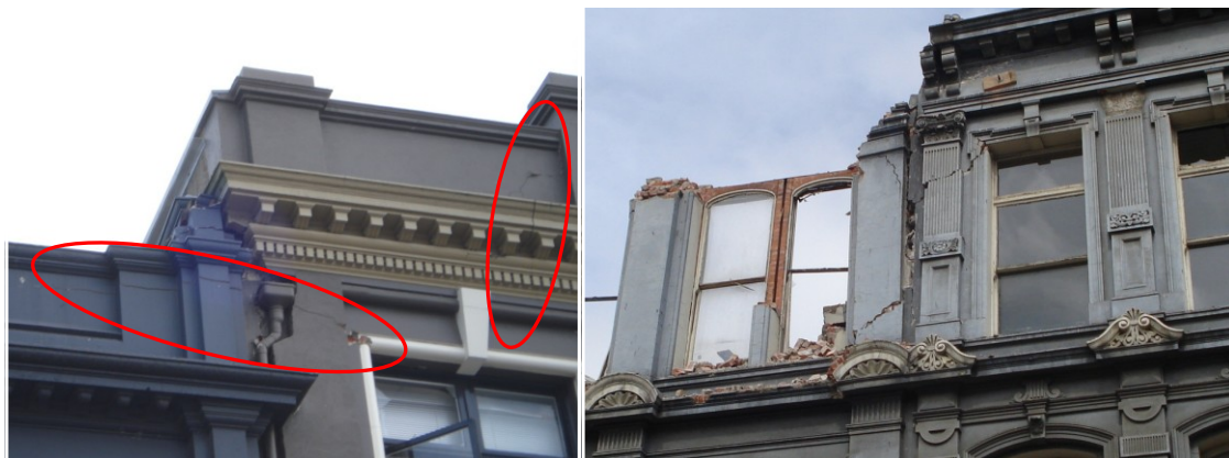
Figure 2.1 Examples of URM pounding damage. Left: minor damage. Right: major damage partially caused by pounding
