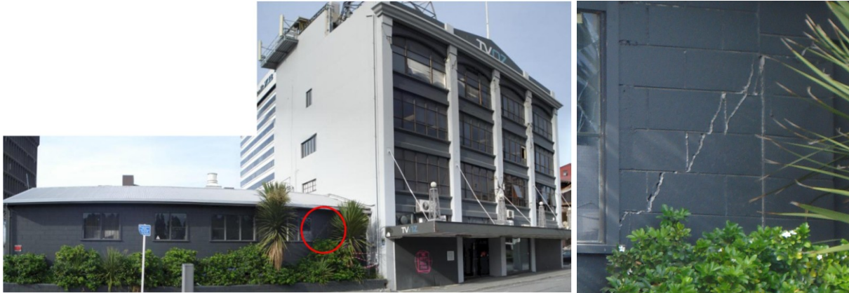
Figure 3.2 Pounding between 1 storey and 4 storey buildings. Damage to four storey building not attributed to pounding
