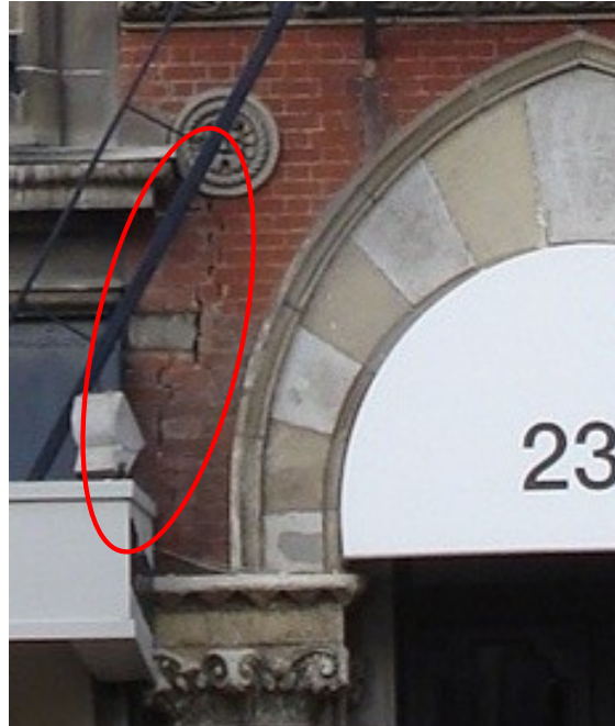
Figure 3.4 Masonry damage after the Darfield earthquake
