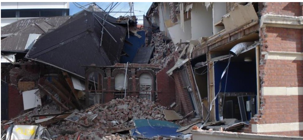
Figure 3.3 Two storey building collapse involving pounding. Primary cause of collapse is attributed to URM construction
