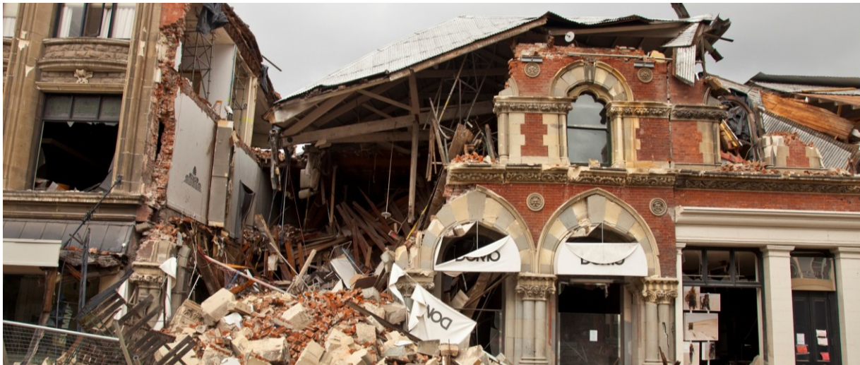
Figure 3.5 Building collapse involving building pounding. Primary cause of collapse is attributed to URM construction. Photo courtesy of Colin Monteath, Hedgehog House
