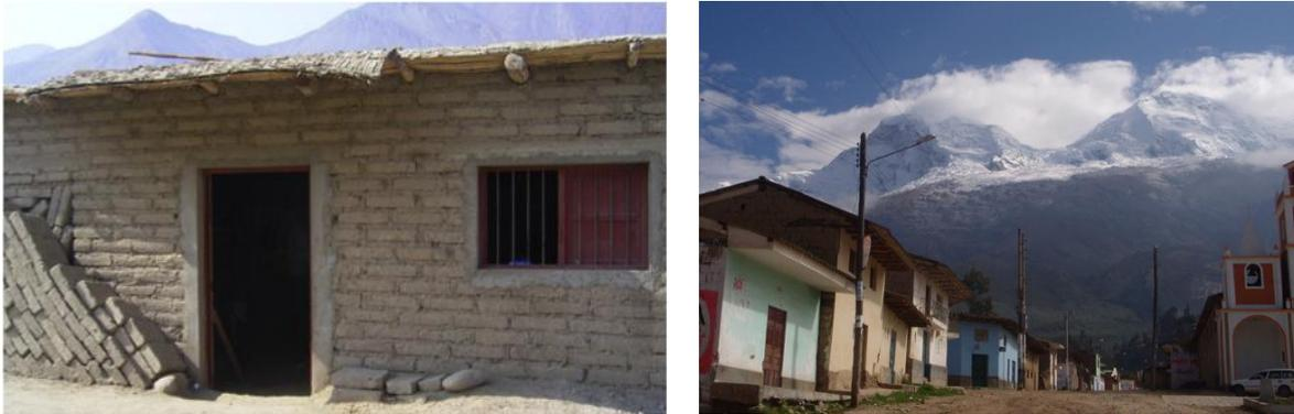
**Figure 2.2.** Single storey adobe residence with woven bamboo roof cover found in the coastal regions of southern Peru (L) and adobe houses with heavier roofs found in the Andean regions of Peru (R)
