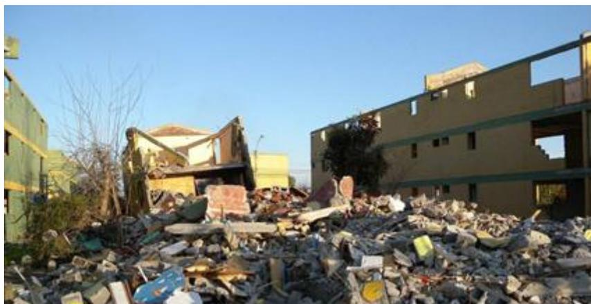
**Figure 2.5.** Collapse of a 3-storey confined masonry building in Santa Cruz (2010 Maule, Chile) earthquake
