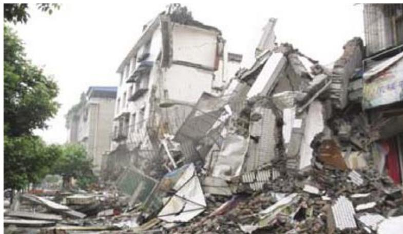
**Figure 2.4.** A 4-storey load bearing masonry failure in Hehuachi District, 2008 Wenchuan. (Zhang and Jin, 2008)
