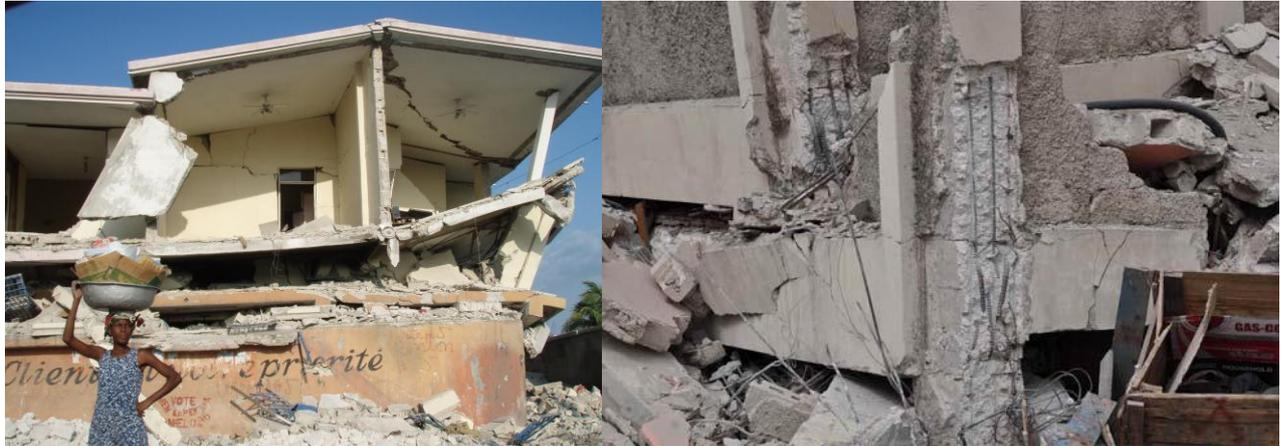
**Figure 2.6.** Typical failure mechanism of three-storey confined masonry buildings in Port-au-Prince; and widespread poor “confinement”, witnessed after the 2010 Haiti earthquake
