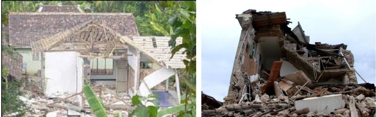
**Figure 2.3.** Partial collapse of load bearing brick masonry buildings (LBM) low rise in 2006 Yogyakarta, Indonesia (L) and mid-rise in 2009 L'Aquila, Italy earthquakes (EEFIT, 2009)
