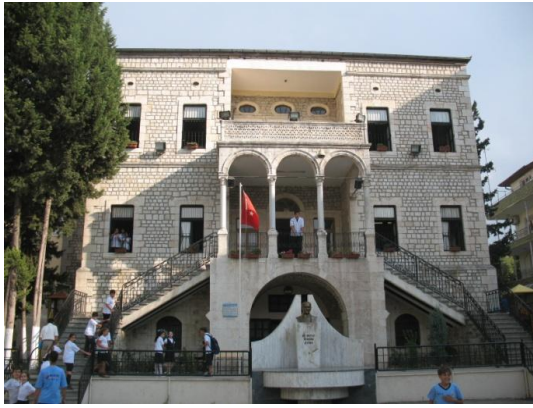
a) View of the instrumented school building
