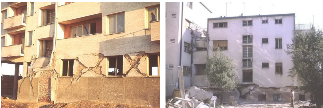
Figure 1.2. Damage on residential masonry buildings after 1963 Skopje earthquake (Ambraseys, 1967)
