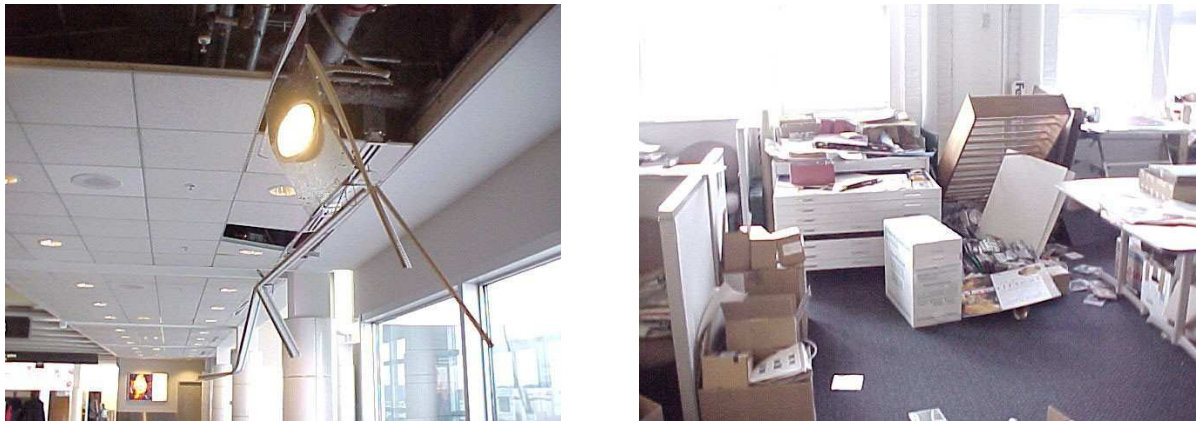
Figure 3. Typical nonstructural damage (Source: FEMA)
