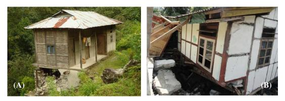
Figure 7. (A-B) Ekra houses, Sikkim from post-earthquake reconnaissance survey (18 September, 2011)
