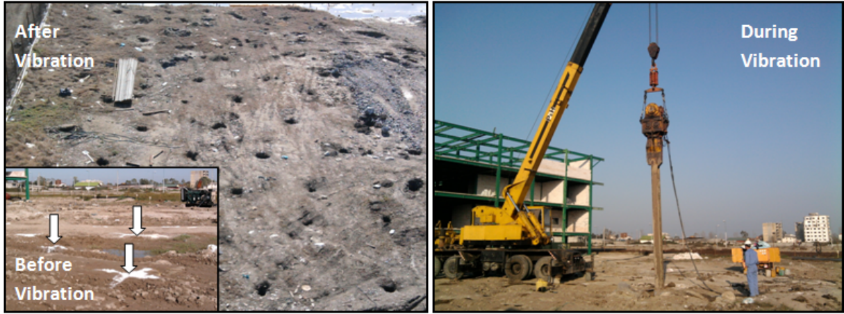
Figure 3.3. After vibrating a pile in the desired depth, the pipe was withdrawn and after outing of the ground, other points were attacked one by one in turn.
