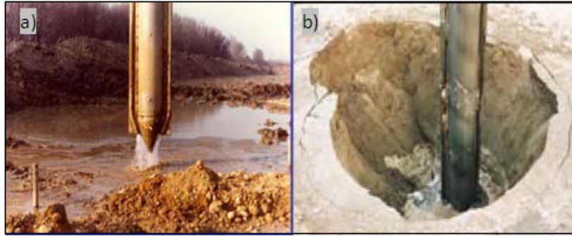
Figure 3.1. Craters with diameters of 3 to 4.5 m (10 to 15 feet) can form around vibrator if backfill is not added. a) Before penetration. b) After penetration. (Keller 2012)
